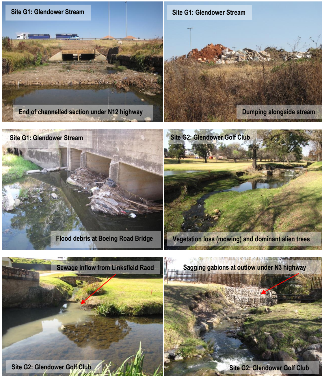
Figure 16. Photographs showing some of the impacts considered in the Index of Habitat Integrity for Glendower Stream.
