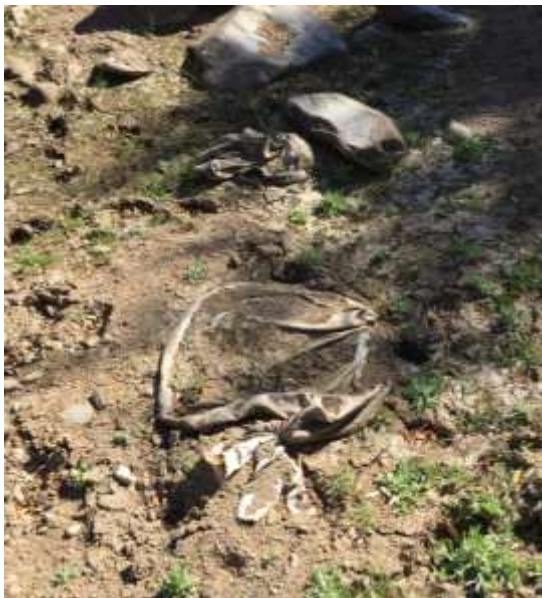
Figure 4.5 Sandbags and pipes used in the clean-up operations of the Meirings River following the diesel spill should be removed from the channel.
