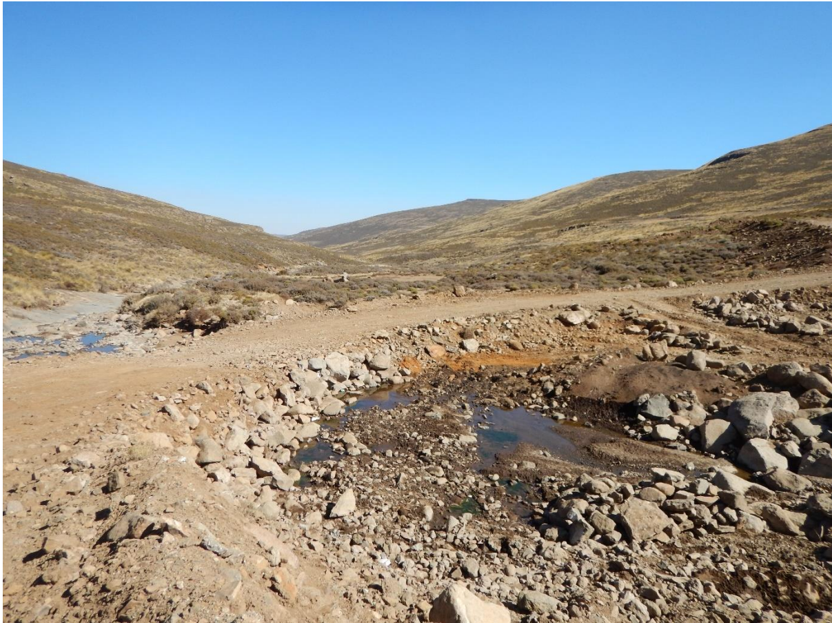
Figure 14: The Mothae River; a road had been constructed across the river channel.
