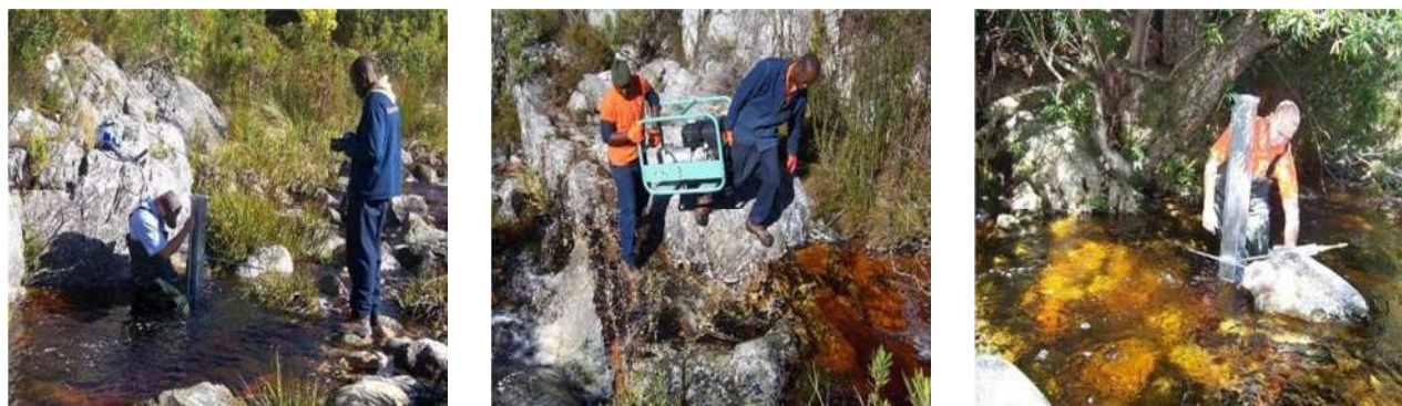
Figure 4.1. Stilling well installation.
