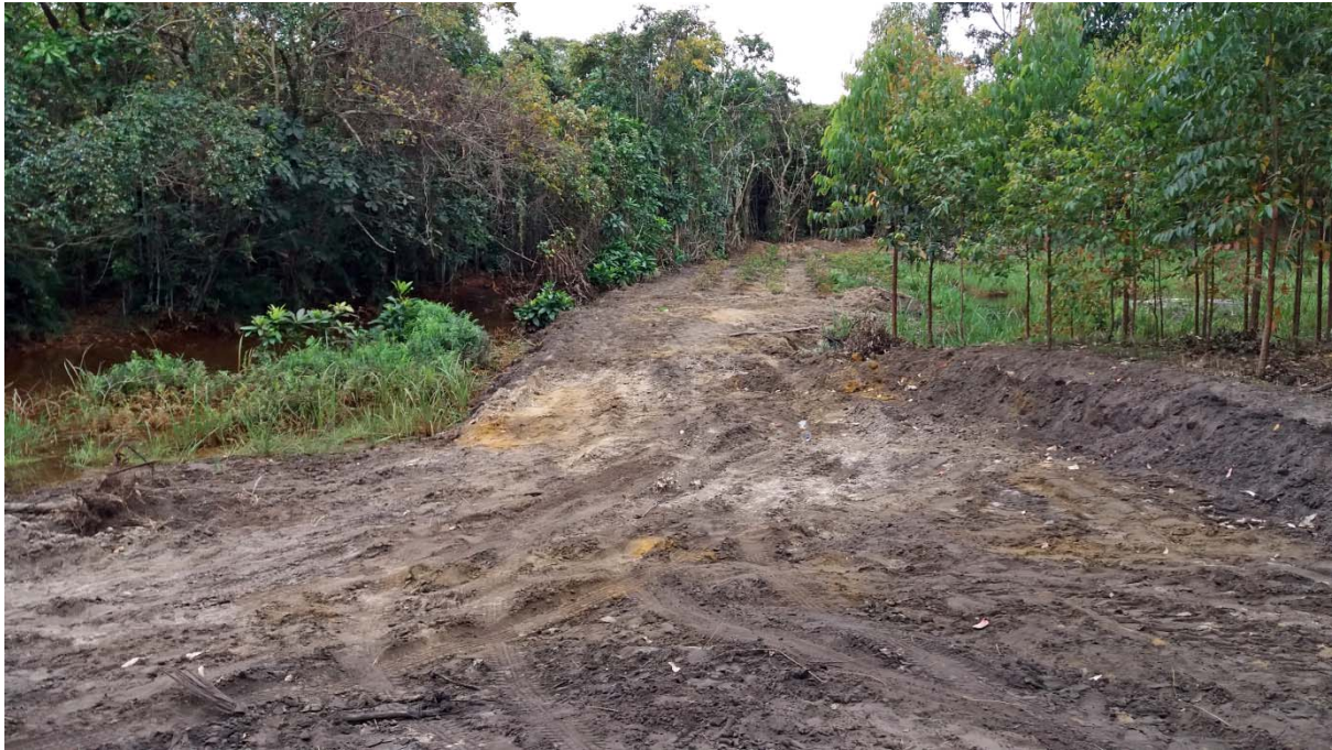
Figure 12 Impacts noted at site 14: view along the river.
